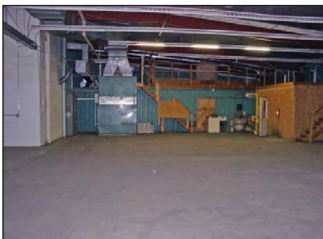
Mezzanine Above Office
